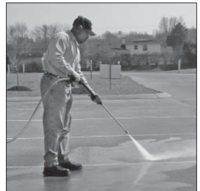
Figure 16 - Optimum angle to cleaning surface
