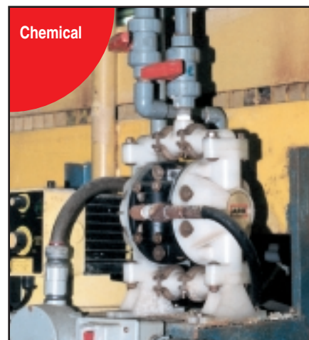
This ARO 666057-444 pumps magnesium sulfate
